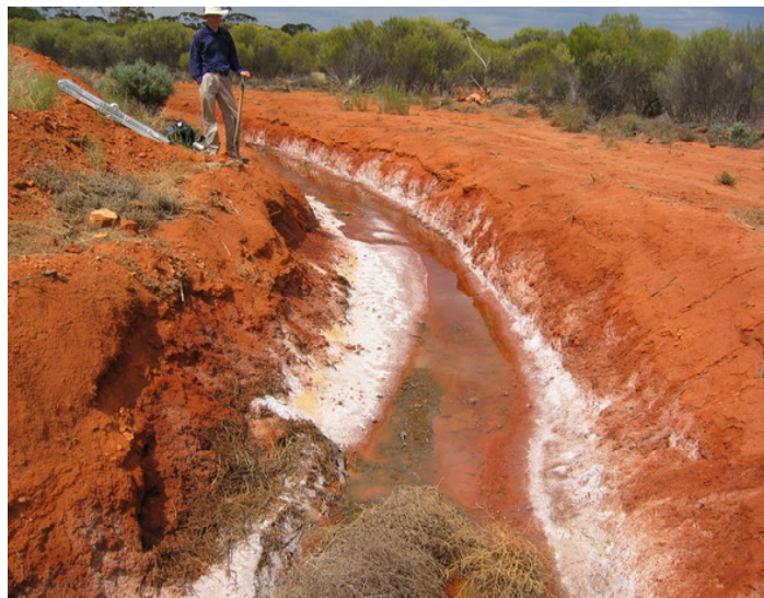
Figure 2. Typical deep acidic saline drain with in the WA Wheatbelt.
