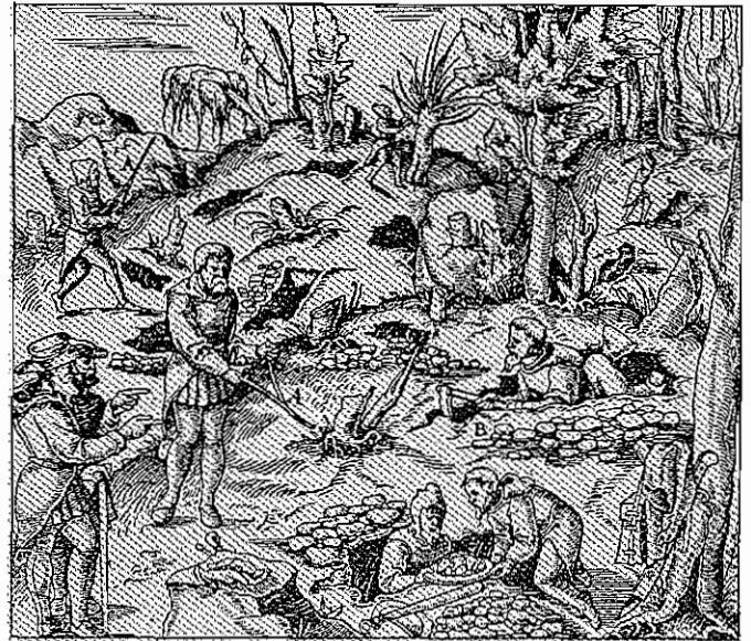
Figure 1. 16th century illustration of the divining rod, from Agricola (1556, p. 40). A is the divining rod, and B shows searching for ore veins by trenching, the method favored by Agricola.
